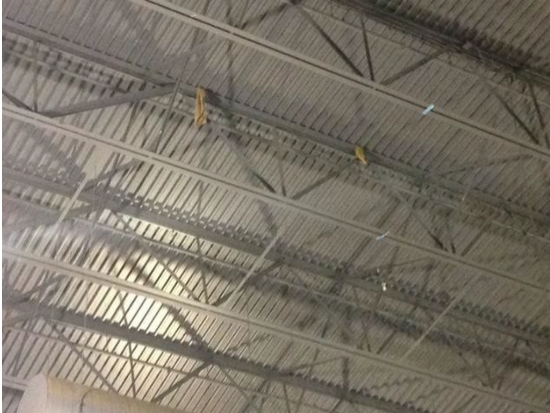
Panel Trusses – located in Halls A, B, C & D – points are rigged where cross bars meet (see where burlap bags are in picture)
