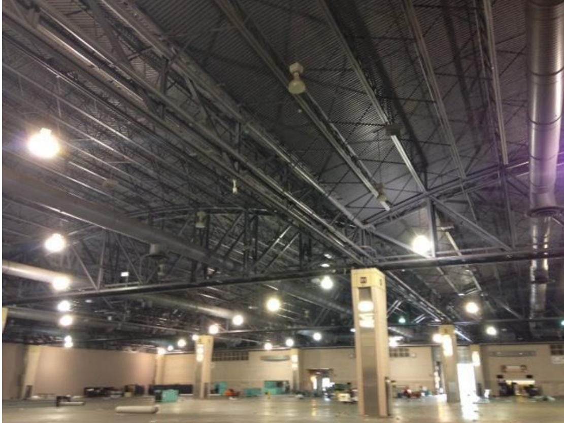
Hall A – as you enter from the concourse
