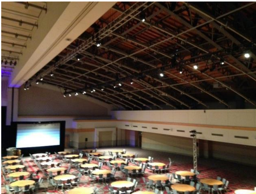
Ballroom A – Ceiling and lighting grid (lighting on truss that is rigged is not permanent part of room)
