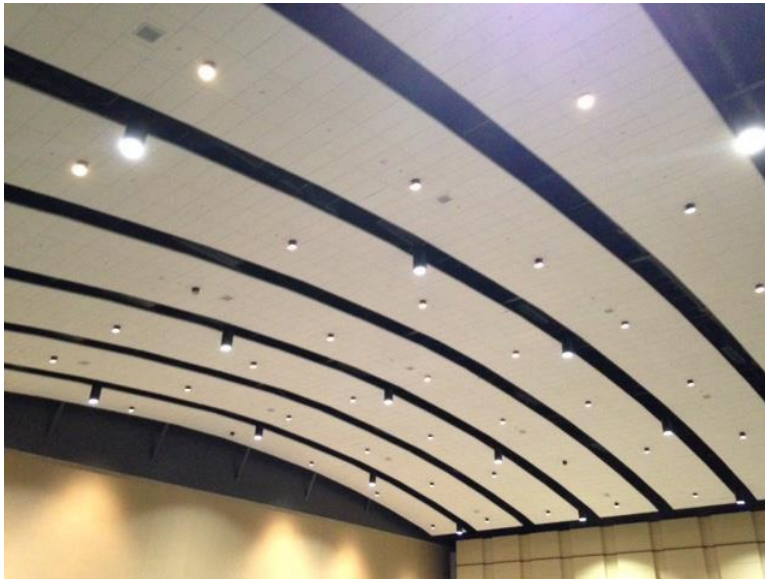
Terrace 4 – Full view of ceiling from corner of room
