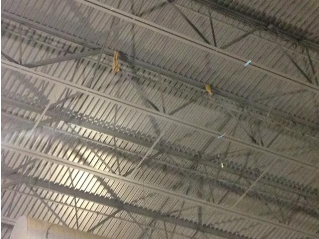
Panel Trusses – located in Halls A, B, C & D – points are rigged where cross bars meet (see where burlap bags are located in picture)
