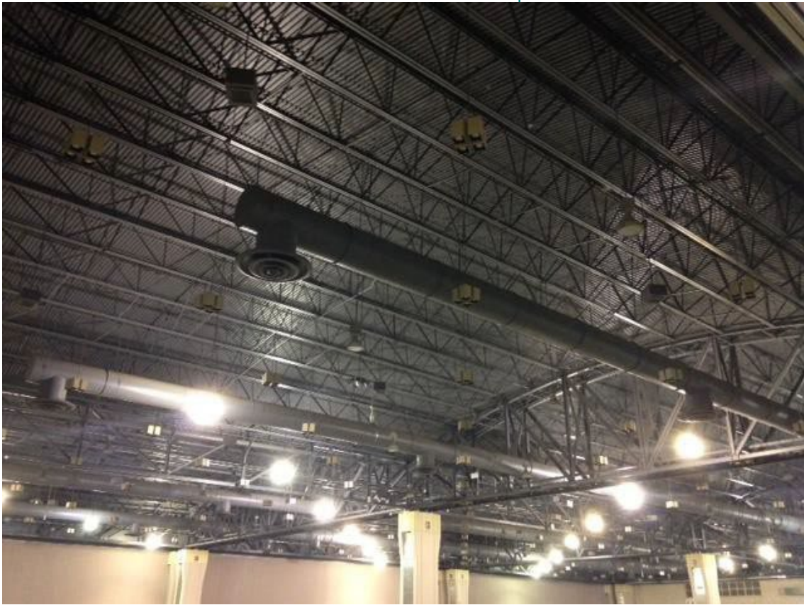
Panel Trusses - Halls A, B, C & D
