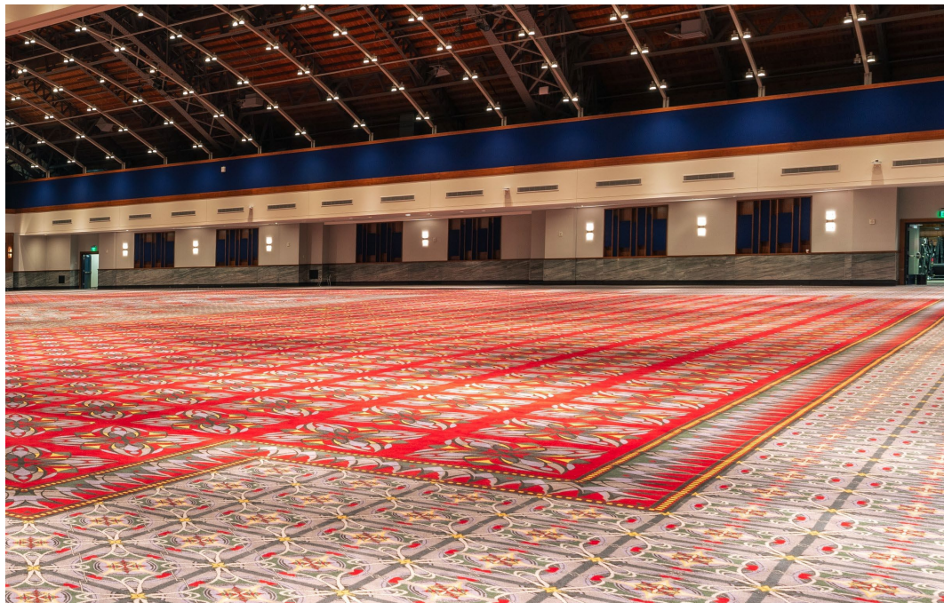
Ballroom A - ceiling and lighting grid
